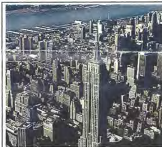
In the first portion of a three-phase retrofit, owners of New York's Empire State Building replaced over 5,000 windows with energy-efficient models that are expected to provide steam and electricity cost savings amounting to almost $1 million a year.
