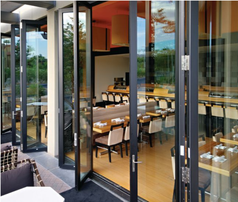
Indoor-outdoor lounge seating at restaurants and hotels is a big draw for customers, and the latest trends in fenestration systems, such as folding doors and window walls, can easily accommodate. The doors at this sushi restaurant in Phoenix leave little distinction between the dining and patio areas.
