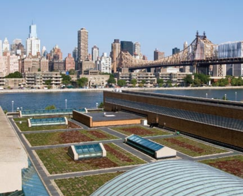
Modular planting trays were chosen for the green roof crowning Con Edison's Long Island City, N.Y., training facility.
