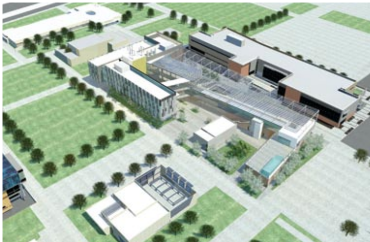
HGA's design for the Los Angeles Harbor College Sciences Complex building combines white reflective roofing and BIPV (building-integrated photovoltaic) systems, which provide some shading, thereby reducing solar heat gain.
