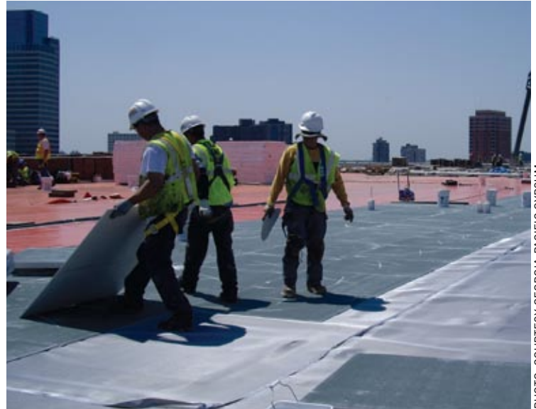
Workers install a new roof on the Target Center, a Minneapolis entertainment arena, the fifth-largest extensive vegetative roof system in the U.S.
