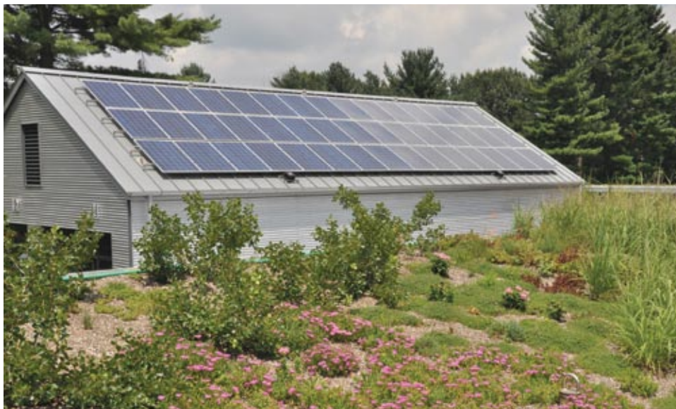
Two green roofs above the garages at the Horticulture Center at the University of Pennsylvania’s Morris Arboretum, designed by Overland Partners Architects, are part of a larger rooftop strategy incorporating PV and a high-reflectance metal roof. Two types of planted roofs, intensive or extensive, are being used in green projects.
