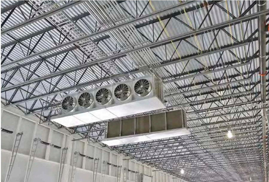
Standard steel joist and deck with engineered efficiencies.
