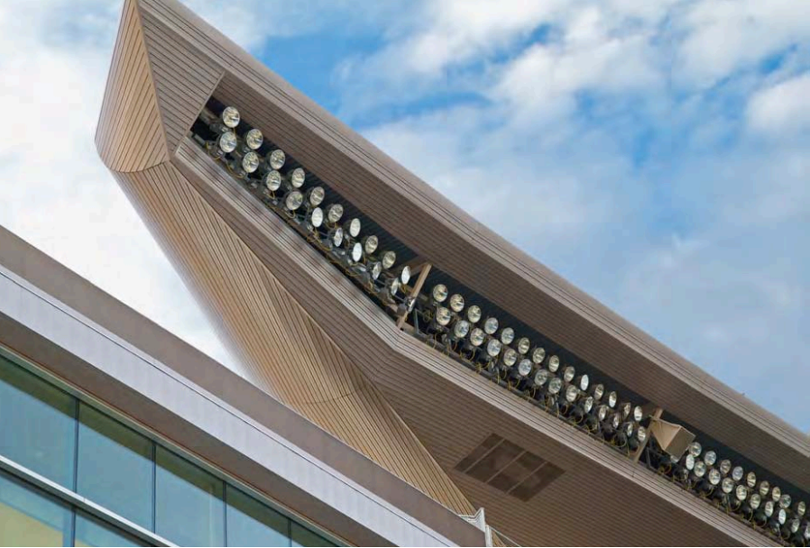
Architectural steel decking with lineal plank aesthetic as stadium cladding.
