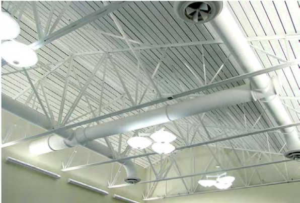
Steel joist and dovetail deck with MEP integration.
