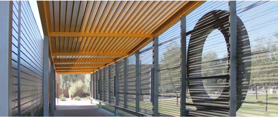
Perforated architectural steel decking for UV protection.
