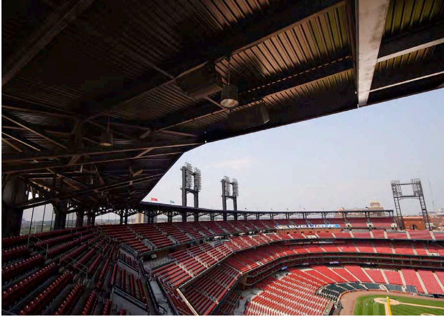
Standard steel joist and deck systems with factory coatings.
