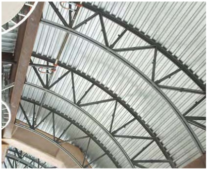
Special profile steel joists and decking for curved entry.
