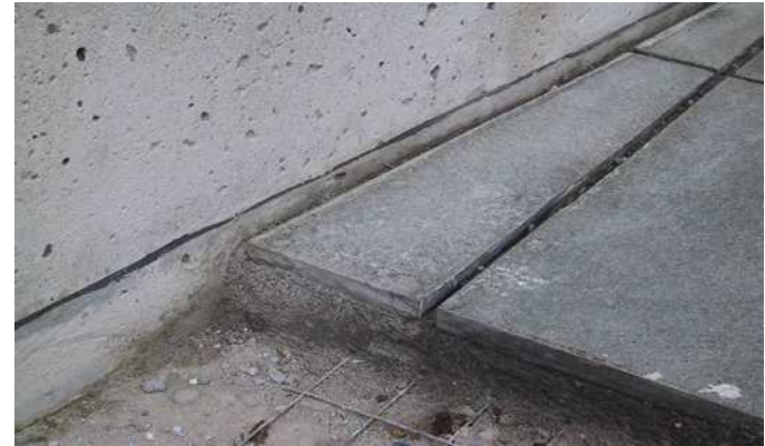
Shown is a large profile stone installed at the perimeter of a room. A movement joint is required where the floor meets the wall.
