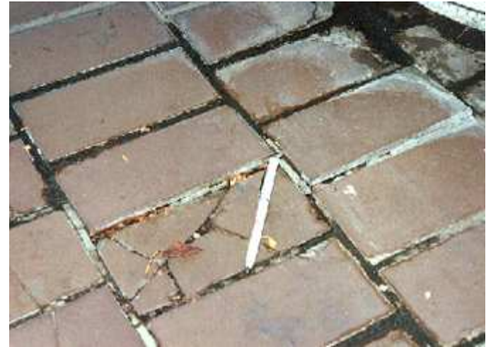
Proper waterproofing design would have saved this installation.
