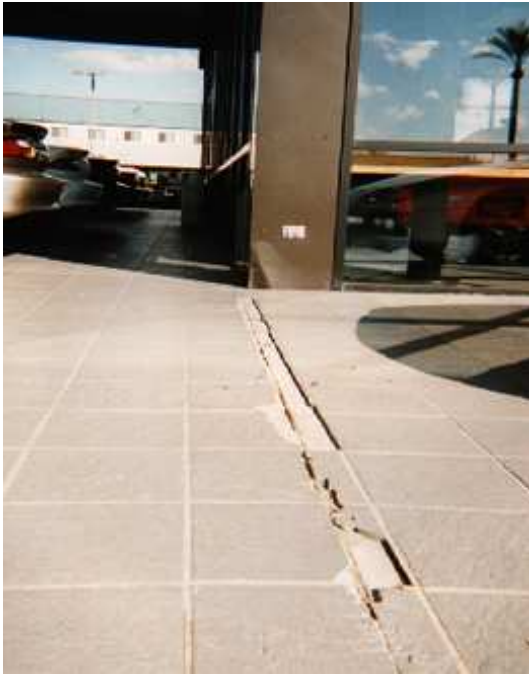
This limestone floor failed as a result of a misplaced soft/control joint.
