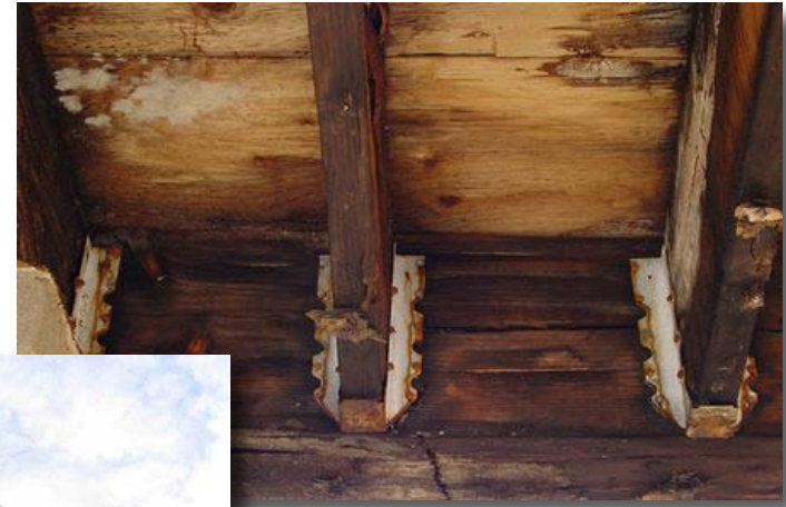
Structural Wood Decay
