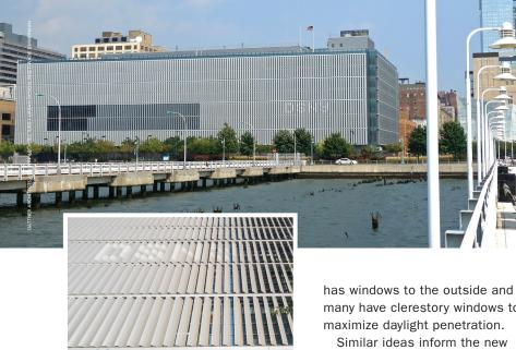
The design for a sanitation garage in Manhattan employed 2,600 custom perforated metal vertical sunshades to mitigate solar heat gain and glare and block vehicle headlights.
