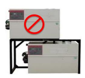
One unit disabled: 50% loss of DHW Tank disabled: 100% loss of DHW
