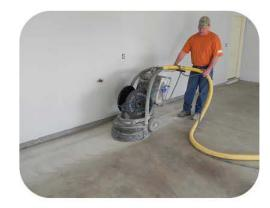
Refer to SSPC SP-13 Surface Preparation of Concrete and ICRI Guideline Number 310.2R industry standards Improper surface preparation is responsible for the majority of coating failures
