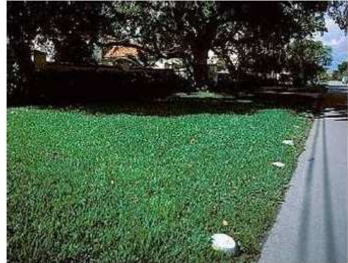
Delineated houlder parking on plastic grass porous pavement
