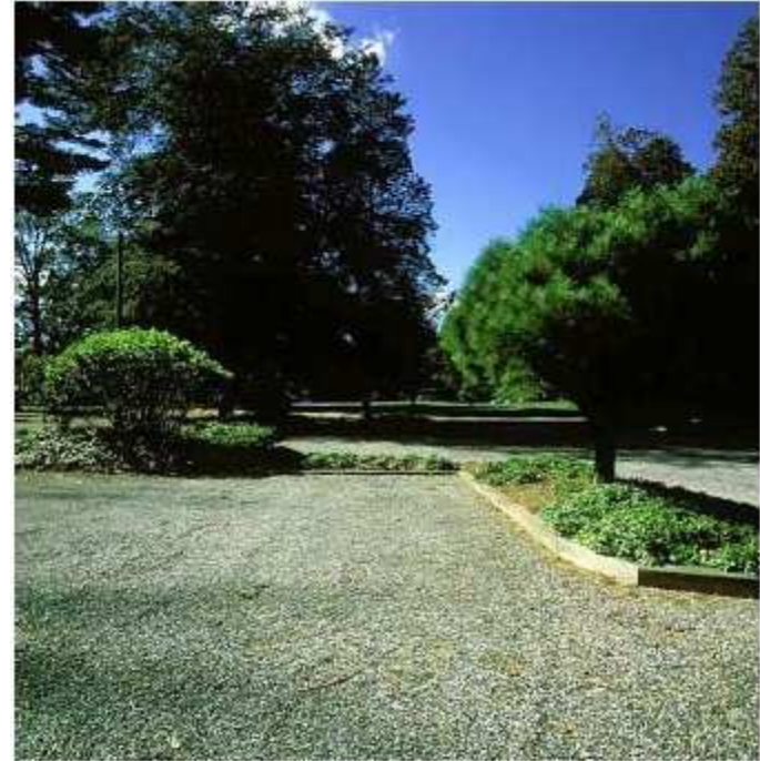
Porous flexible gravel paver parking lot.
