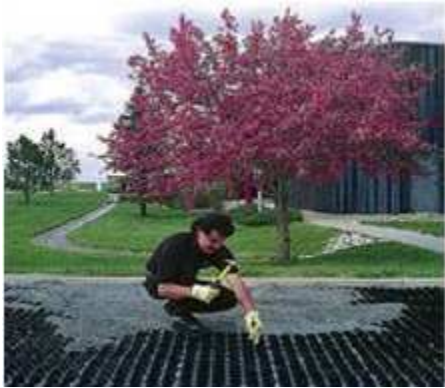
Secure base with connectors
