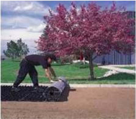
Unroll paver, connect and cut as needed
