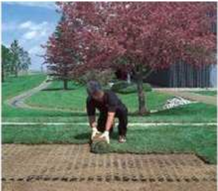
Lay sod or seed with mulch
