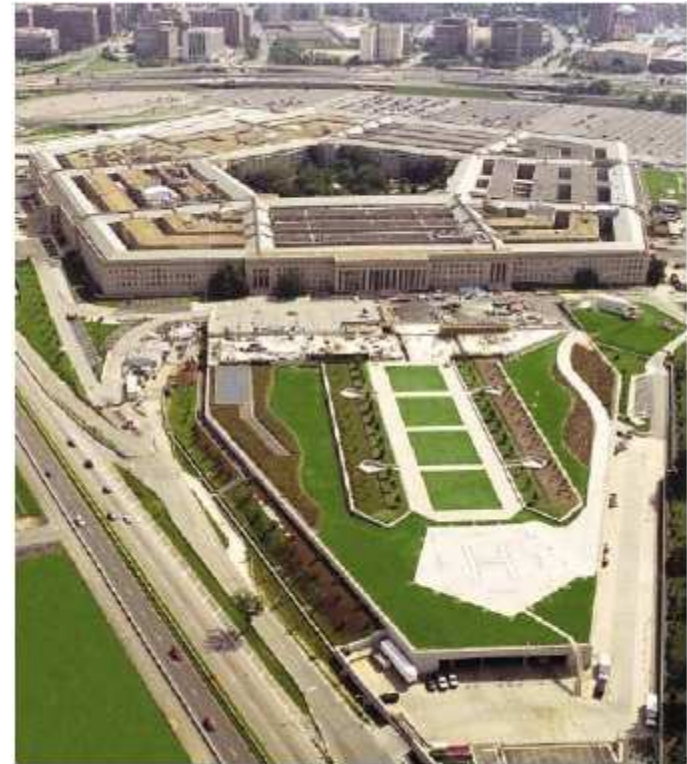
Grass porous pavement on the Pentagon Remote Delivery Facility (RDF), Arlington, VA
