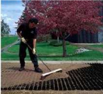
Fill rings with clean sharp sand
