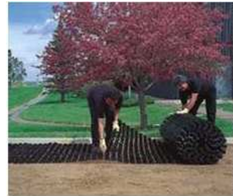
Roll out flexible, grid
