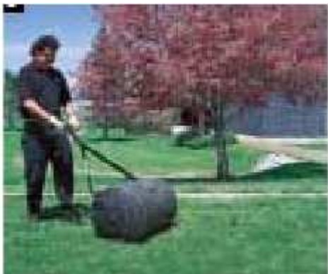
Roll sod with heavy roller
