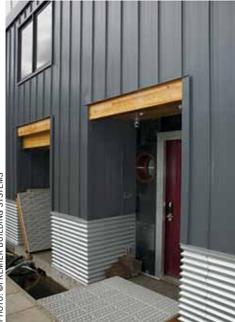
Structural insulated panels in a multifamily project in Seattle. The high strength and low weight of SIPs are ideal for use with standing-seam metal cladding.
