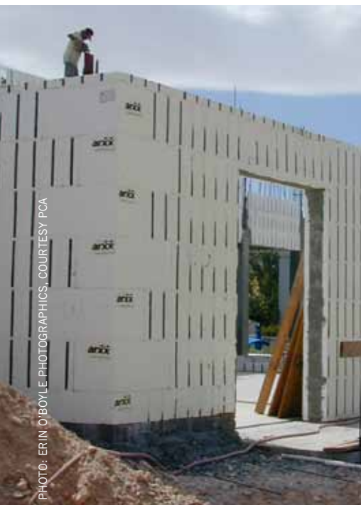
Insulating concrete forms (ICFs) can serve as essential building blocks for creating airtight, energy-efficient enclosures and are compatible with most types of cladding.
