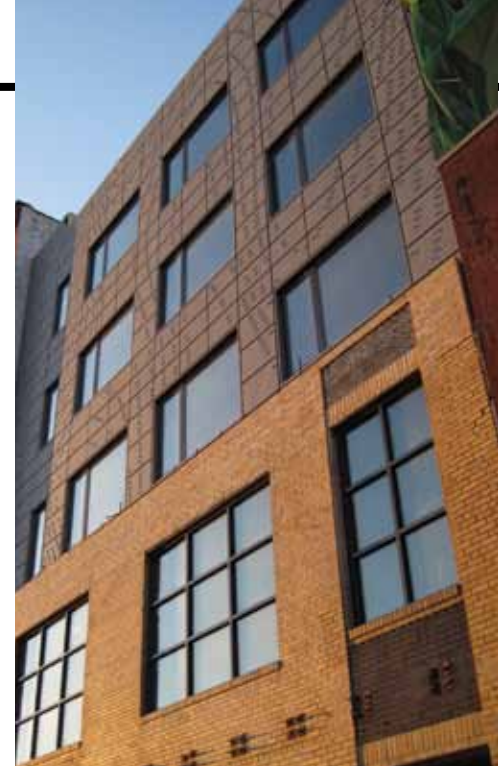
Zinc rainscreen façade added decorative patterning and rhythm to an infill structure above a contrasting brick veneer. Rainscreens can be used for overcladding existing buildings with moisture infiltration problems.
