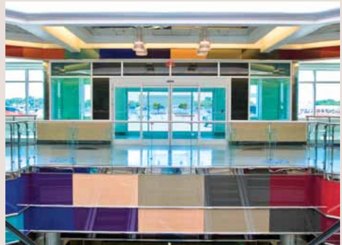
Automatic door installed at the Kansas City airport. The door shown here (DORMA ESA200 model) is an extruded aluminum stile and rail door designed for interior or exterior applications where emergency breakout of only the sliding panels is required. In general, automatic doors provide a common solution for meeting ADA requirements.
