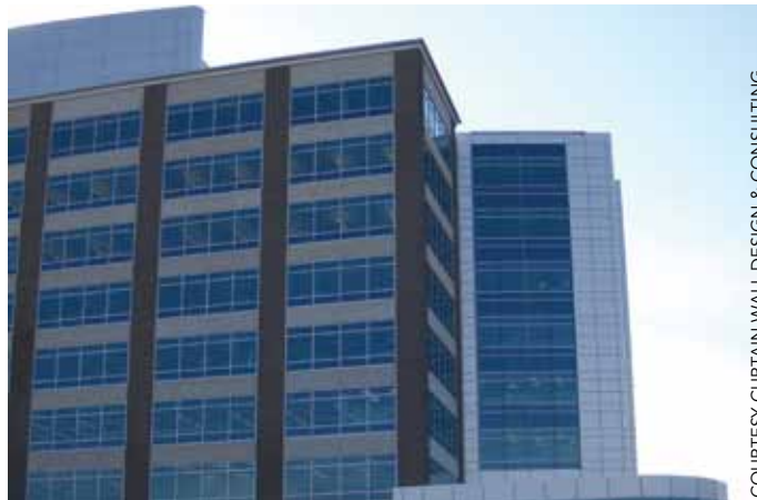
This pre-assembled, factory-glazed window wall system, which offers enhanced quality control, was installed in precast concrete openings.
