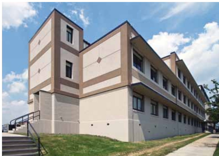
Overcladding existing masonry walls with rainscreens or barrier wall systems (as shown in this before-and-after sequence) is an effective way to provide improved thermal performance and resistance to air and moisture infiltration.
