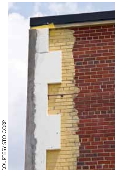
Overcladding existing masonry walls with rainscreens or barrier wall systems (as shown in this before-and-after sequence) is an effective way to provide improved thermal performance and resistance to air and moisture infiltration.
