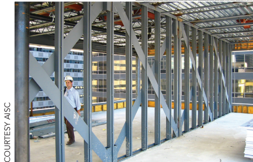
The Harman Group (SE) combined load-bearing steel wall panels with composite joist floors. This added eight stories and 68,000 sf to the original five-story concrete frame footprint of 2040 Market Street, Philadelphia.
