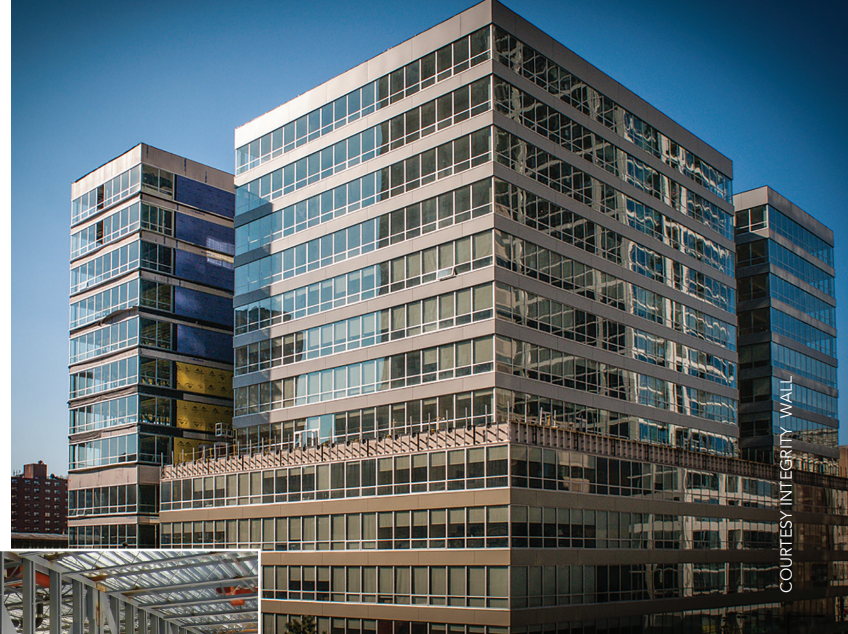
The Harman Group (SE) combined load-bearing steel wall panels with composite joist floors. This added eight stories and 68,000 sf to the original five-story concrete frame footprint of 2040 Market Street, Philadelphia.
