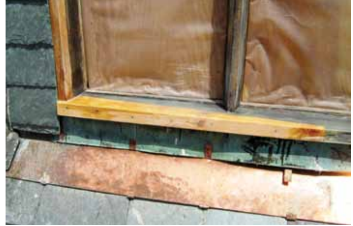
Wood frames too badly deteriorated for consolidation or surface treatments may be restored using a so-called “Dutchman” repair, whereby rotted wood is cut out and a new piece of wood is spliced in its place. Proper treatment often depends on the availability of a skilled carpenter to construct the parts.
