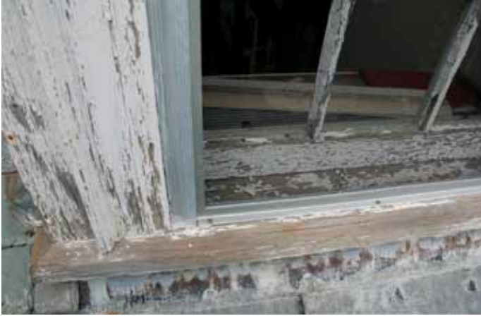
Wood frames too badly deteriorated for consolidation or surface treatments may be restored using a so-called “Dutchman” repair, whereby rotted wood is cut out and a new piece of wood is spliced in its place. Proper treatment often depends on the availability of a skilled carpenter to construct the parts.
