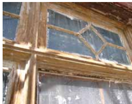
Before, during, and after photos show the restoration of historic wood windows. Strategies may include removal of flaking paint, consolidation or patching of weathered surfaces, and treatment with water-resistant material. Local and state regulations for acceptable materials and details vary widely, so check with the authorities.
