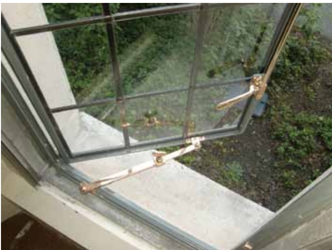
Mockups of proposed window restoration or replacement designs permit on-site evaluation of hardware, operability, aesthetics, and performance.
