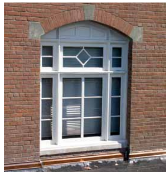
Before, during, and after photos show the restoration of historic wood windows. Strategies may include removal of flaking paint, consolidation or patching of weathered surfaces, and treatment with water-resistant material. Local and state regulations for acceptable materials and details vary widely, so check with the authorities.
