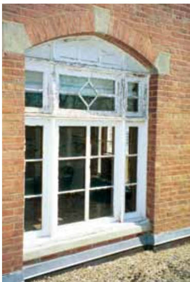
Before, during, and after photos show the restoration of historic wood windows. Strategies may include removal of flaking paint, consolidation or patching of weathered surfaces, and treatment with water-resistant material. Local and state regulations for acceptable materials and details vary widely, so check with the authorities.
