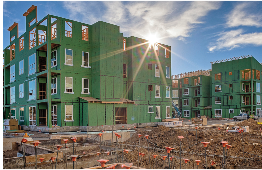
Integrated sheathing and tape systems help protect against air leakage while allowing sufficient vapor permeability.
