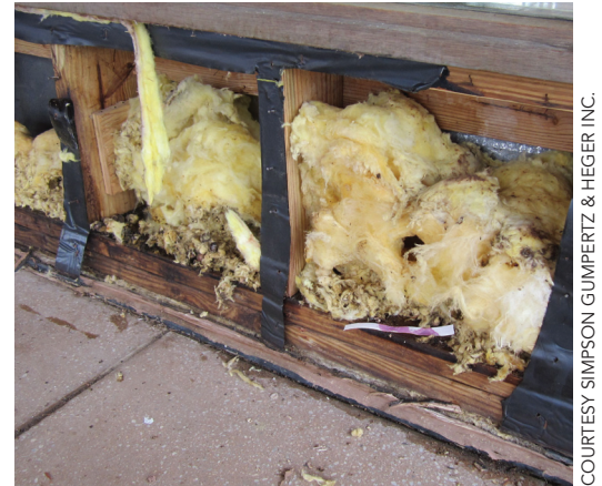
Pictured: moisture-related damage to insulation and wall framing due to the vapor retarder having been installed—improperly—on the “cold” side of wall insulation.
