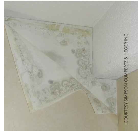
Photo shows mold growth behind vinyl wallpaper due to moisture migration in a structure in a hot and humid climate.
