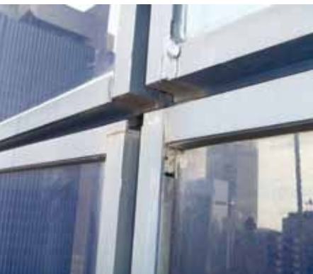
Gaps at frame corners.
