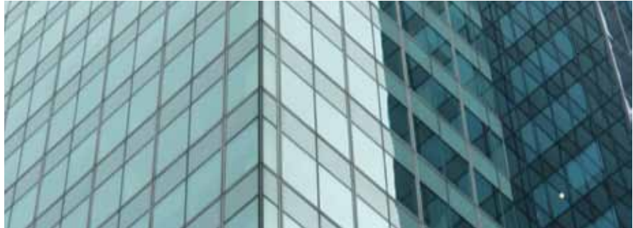
To achieve optimal performance for a well-designed glazed curtain wall., Building Teams should identify emerging problems and take swift corrective action, say the expert authors.
