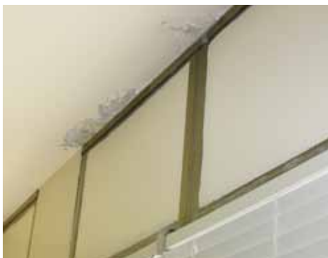
Leaks and drafts in curtain wall assembly.
