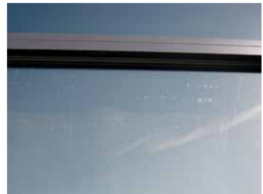
Scratches and hairline cracks.
