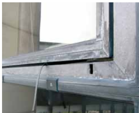
Loose or missing weather stripping.
