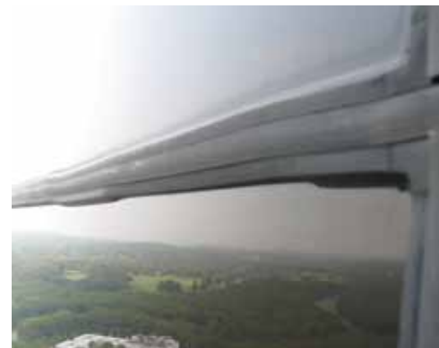
Gaskets disengaged from glazing.
