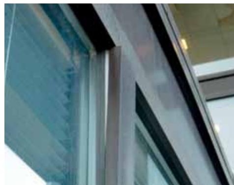
Displaced mullion covers.
