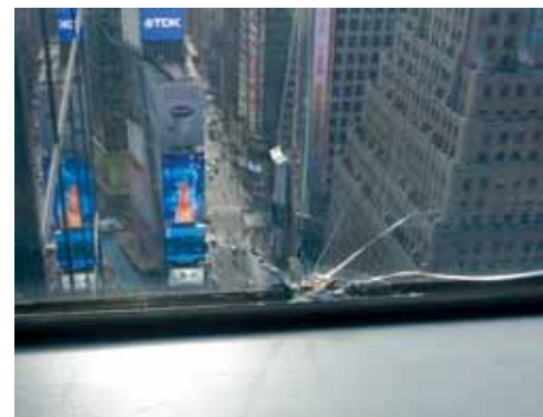
Broken glass in glazed curtain wall.
