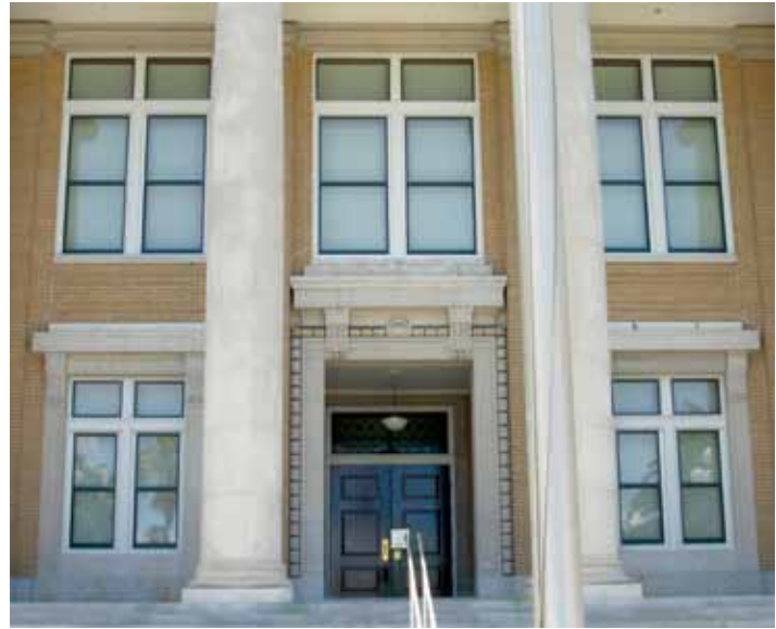
For a 1917 courthouse building in Clearwater, Fla., new replacement windows match the profiles of the original windows while meeting code requirements for hurricane hazards. The deep metal profile (left) is designed to resist thermal bridging.
