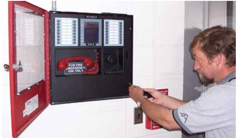
This central panel serves as the backbone for an integrated fire protection and mass notification system at St. Joseph's Hospital Health Center, Syracuse, N.Y. This technology has moved to up to a new level, known as emergency communications systems.
