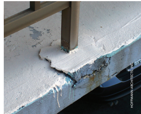
↑ Railing corrosion causing cracks and spalls at post-slab interfaces.
