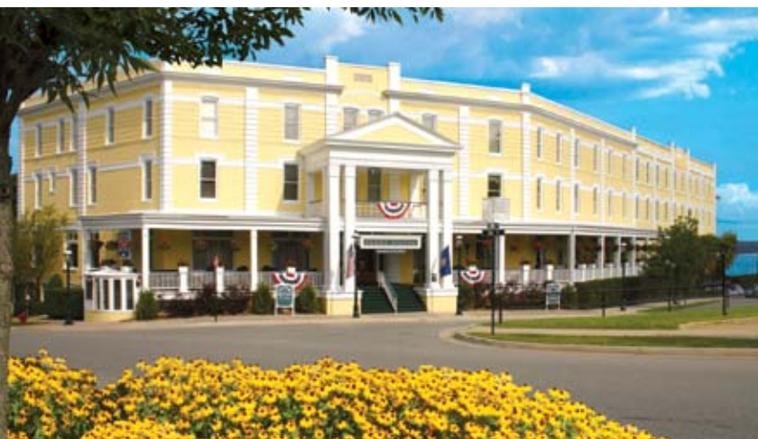
A recent hotel renovation and repaint of the Stafford's Perry Hotel in Petoskey, Mich., employed a smooth high-build coating (from Sherwin-Williams) and a conditioner to address problems of rotted wood, spalling bricks, and peeling paint on the 1899 brick façades.
