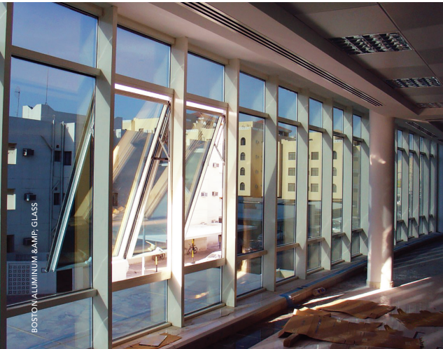
Curtain wall with hopper-style window by Boston Aluminum & Glass, part of a structural glazing curtain-wall system.
