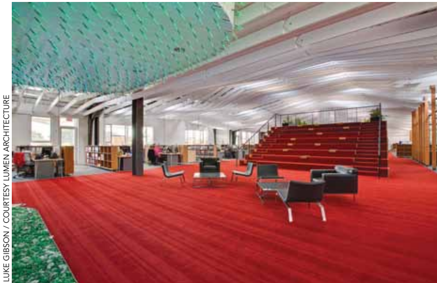
For the Claremont University Consortium renovation, a dropped ceiling plane consisting of felt-wrapped baffles conceals mechanical equipment, including lighting infrastructure. Solar tubes and efficient fluorescent fixtures were arrayed above the baffles in open office space to create an ebb and flow of daylight, via precise controls tied to the BMS. The LEDs in the ceiling are also used on some walls in this project, and can morph from green to blue in response to motion sensors. Early mock-ups and computer visualization informed the design.
