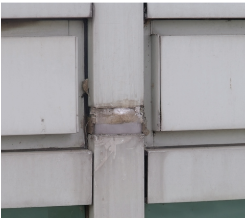
Top: Displaced stone or masonry point to insufficient provisions for material movement. Bottom: Metal cladding displacement and exposure of underlying structural steel.
