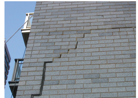
↑ Top: Restrained movement and unforeseen dimensional changes can lead to hazardous displacement conditions. Middle: Cracks at foundation-cladding interfaces. Bottom: Brick expansion leads to vertical and step cracking as forces seek pathways to relief.
