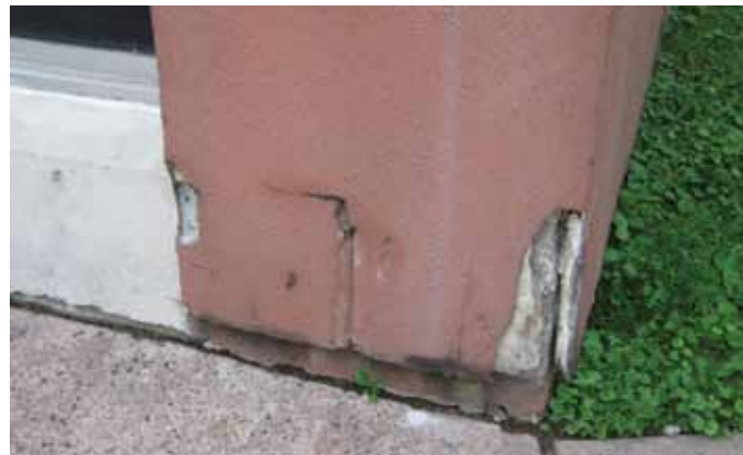
Impact damage that is not repaired promptly provides a pathway for leaks.
