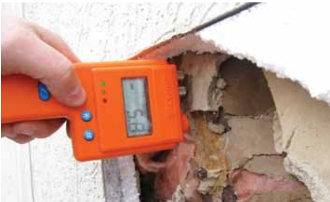
Moisture meters may be used as part of an EIFS failure investigation.
