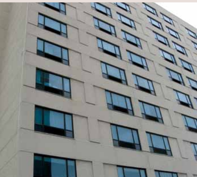
By providing continuous thermal insulation, EIFS can be an energy-efficient wall cladding option.
