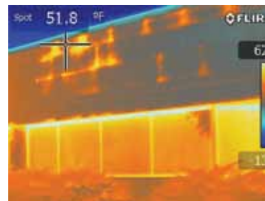
This infrared thermographic scan reveals trapped moisture at insulation board joints.
