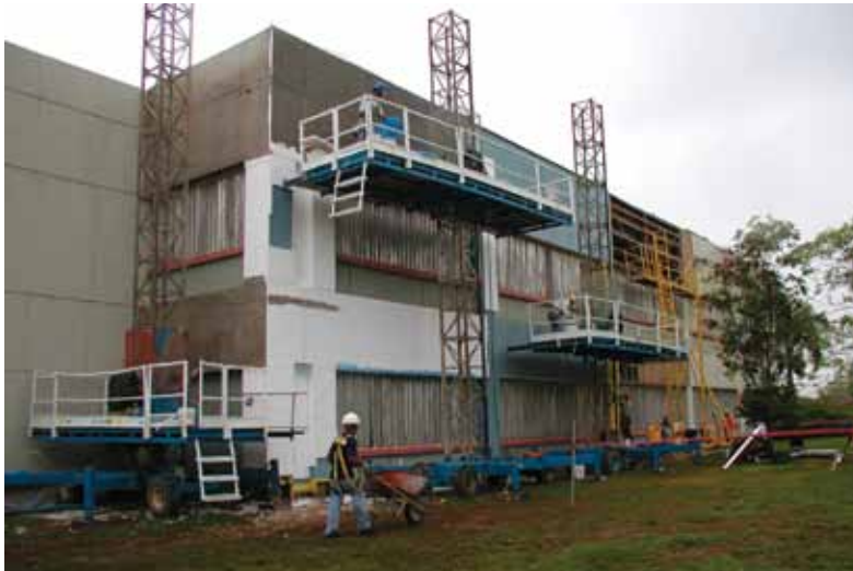
For retrofit projects aiming to improve performance and update appearance, EIFS wall assemblies provide a practical option.
