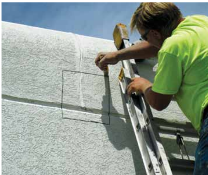
Invasive probes, including test cuts of existing EIFS cladding, can uncover hidden deterioration conditions. A seemingly impervious exterior may mask wet or crumbling wall board beneath the surface.
