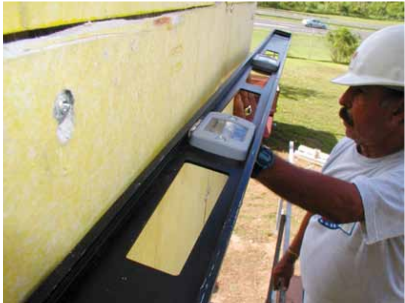
To true the wall surface, the installer should level the insulation board, rather than build up the base coat. Checking stud alignment prior to substrate installation is recommended.
