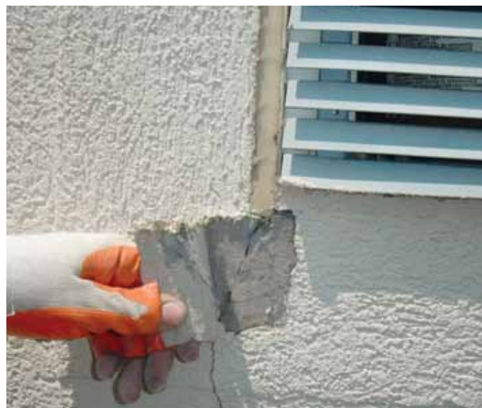
At the corners of windows, doors, and louvers, EIFS design should incorporate butterfly reinforcement, with diagonal pieces of mesh that provide additional reinforcing and prevent cracking.
