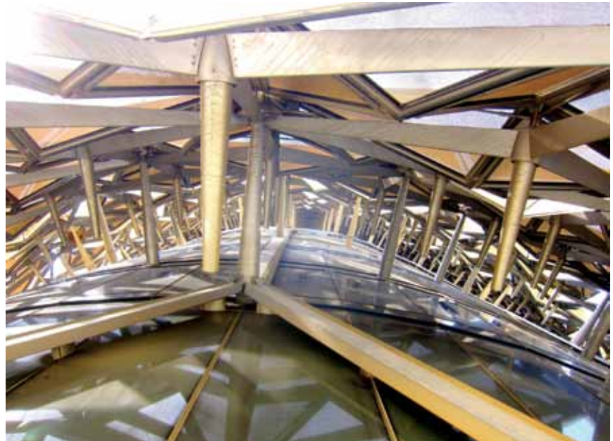
A section view of the Abu Dhabi Investment Council project (also known as the Al Bahar Towers) shows how the translucent shading panels are affixed to the façade. Linear actuators are programmed to open and close each panel based on well-known local climate patterns.
