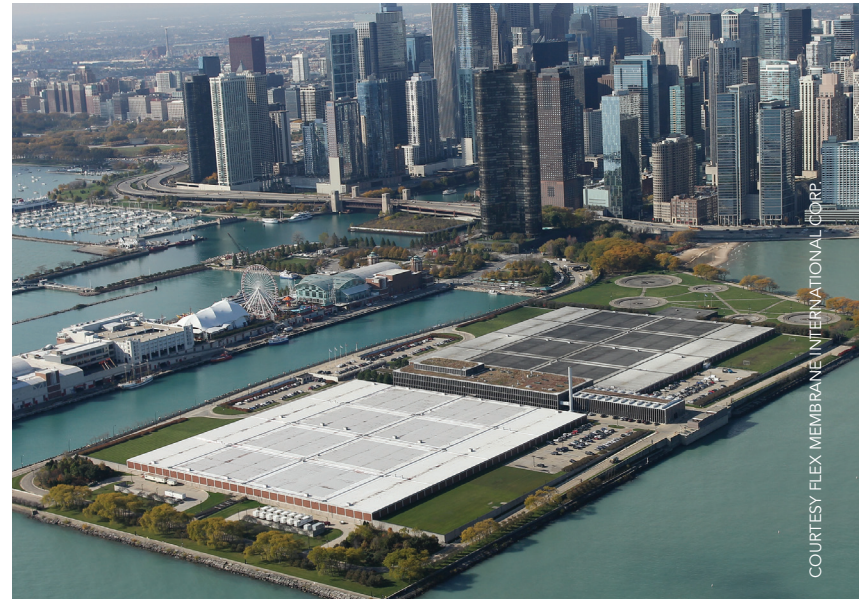
The 10.3-acre reroofing of Chicago's Jardine Water Filtration Plant replaced a 50-year-old tar pitch roof with gravel ballast and 712,000 board-feet of two-inch cellular glass insulation atop 30,000 precast concrete roof channels, capped with KEE thermoplastic membrane.
