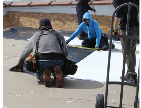
The Red Wing Shoe roofing team chose a flexible TPO membrane to ease installation and flashing details, using heat-welded rather than taped seams.
