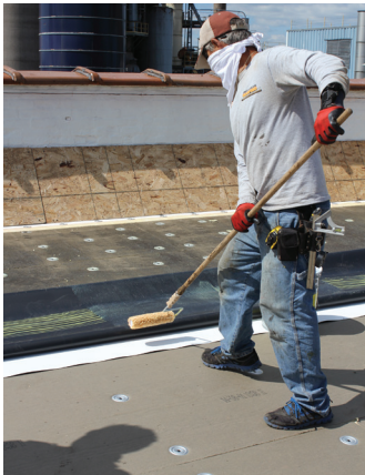
The Red Wing Shoe roofing team chose a flexible TPO membrane to ease installation and flashing details, using heat-welded rather than taped seams.
