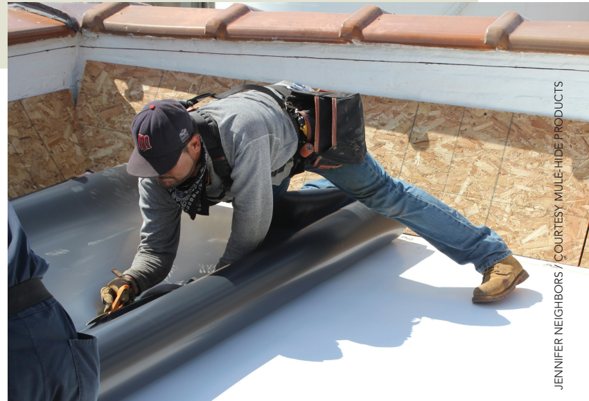
Reroofing the Red Wing (Minn.) Shoe Company's facility with a 60-mil white TPO membrane and heat-welded seams over polyiso insulation.
