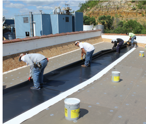
The Red Wing Shoe roofing team chose a flexible TPO membrane to ease installation and flashing details, using heat-welded rather than taped seams.
