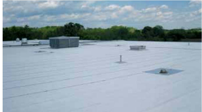
Incorporating a light-colored cap sheet with a high SRI into a traditional modified bitumen roof system can improve energy performance.
