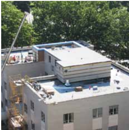
Roof replacement at a suburban or rural location may involve the use of a crane to facilitate delivery of materials.
