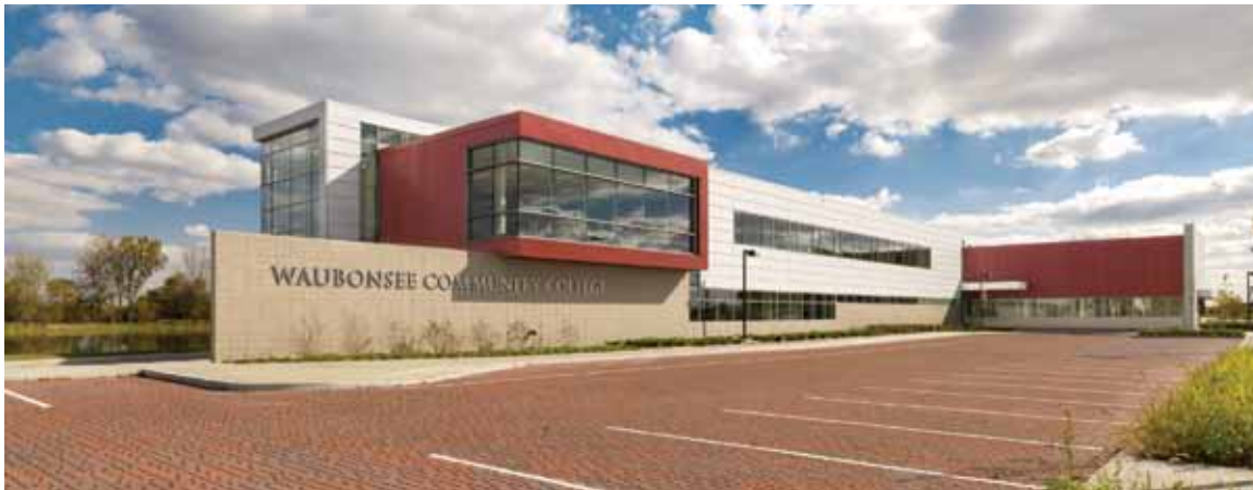
Waubensee Community College in Plano, Ill., chose a metal panel system coated with a protective white polyvinylidene fluoride (PVDF) resin-based finish. The architect for the 33,000-sf project was Holabird & Root.
