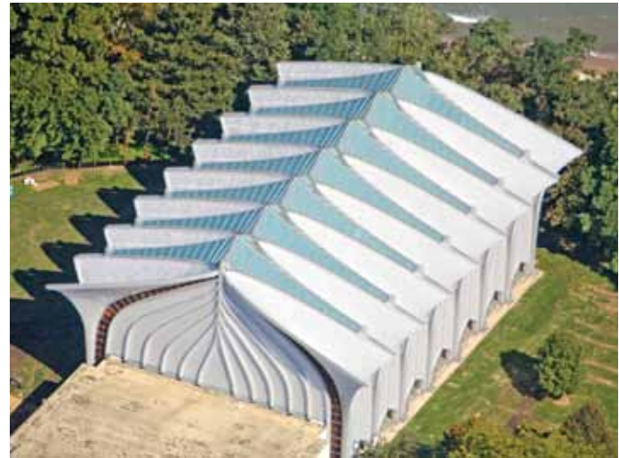
The roof of the North Shore Congregation Israel synagogue in Glencoe, Ill., is treated with a polyvinylidene fluoride (PVDF) coating that reduces solar heat gain and UV emissivity to create a cool roof.
