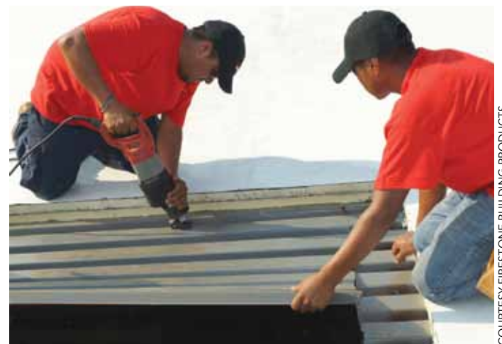
COURTESY FIRESTONE BUILDING PRODUCTS
