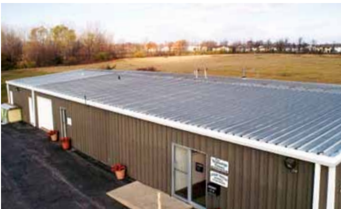
Before-and-after of a retrofit project in Saginaw, Mich., where a single-ply membrane was installed over an old structural metal deck. Such roof retrofits can protect buildings against rain and snow, ice buildup, rust, and corrosion. Such systems can be preabricated in a factory, saving labor costs.
