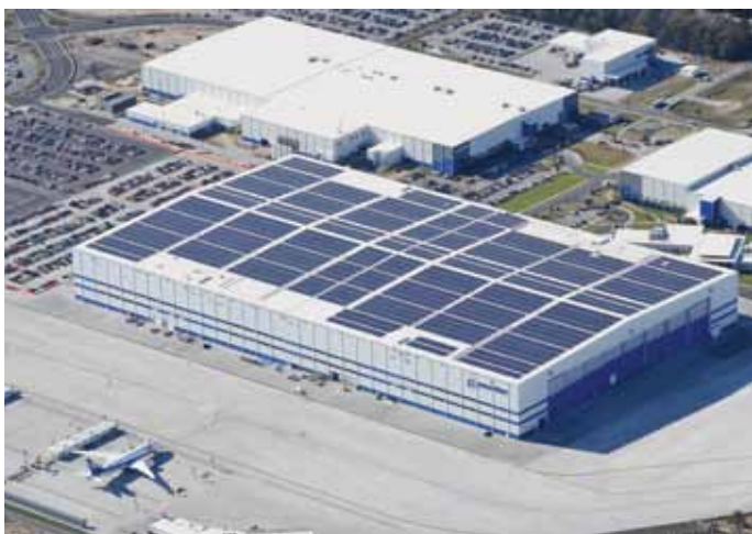
One of the largest PV installations in the country, thin-film solar laminate panels on the roof of South Carolina's 1.2-million-sf Boeing 787 Final Assembly Building are providing the site with 2.6 MW of power.
