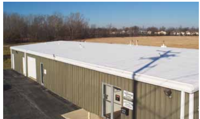
Before-and-after of a retrofit project in Saginaw, Mich., where a single-ply membrane was installed over an old structural metal deck. Such roof retrofits can protect buildings against rain and snow, ice buildup, rust, and corrosion. Such systems can be preabricated in a factory, saving labor costs.
