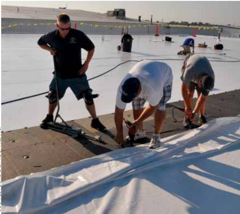
COURTESY DURO-LAST ROOFING, INC.
