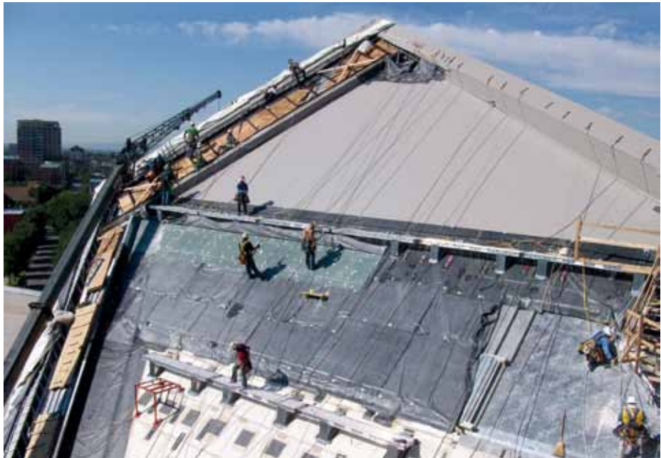
Crews from Black Roofing, Boulder, Colo., work on a 10/12 slope to apply an 80-mil PVC membrane to the roof of the Denver Art Museum, designed by Daniel Libeskind. The original titanium roof started leaking soon after completion in 2006. The job took 31 roofers seven months to complete.
