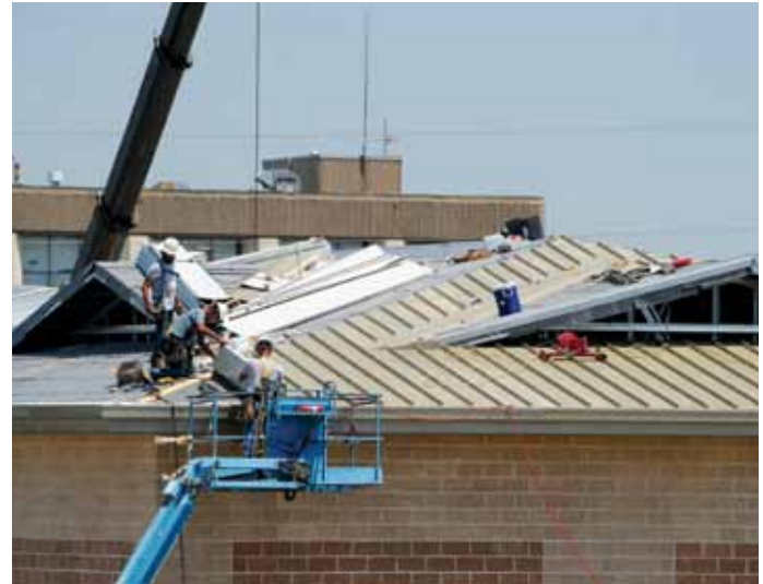
Roofing contractors from Compass Building Systems, Dallas, work on the retrofit of the roof at the Dallas County Water Treatment Facility. Such retrofits can address problematic water discharge and other roof issues.
