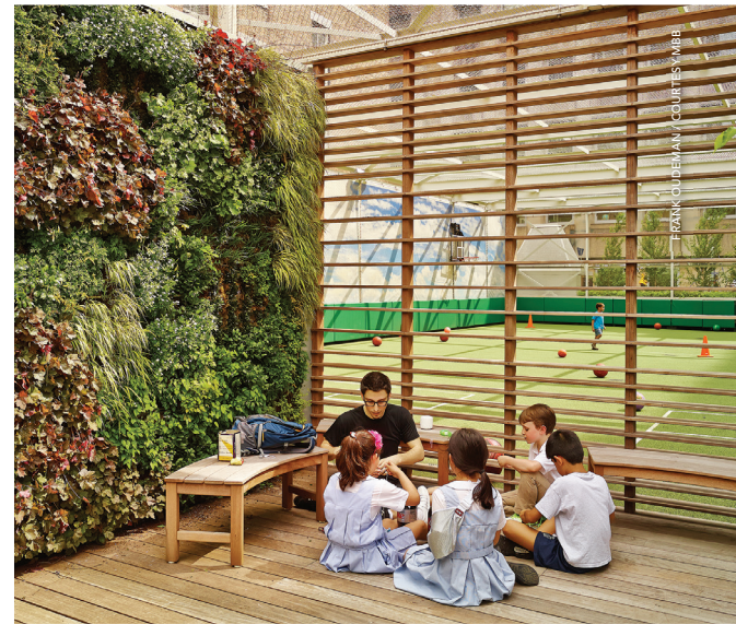
↑ The rooftop deck at St. Hilda’s and St. Hugh’s has an adjustable pedestal deck, rubberize flooring, protective fencing, and extensive plantings, including a living wall.
