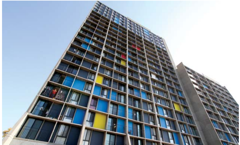
Skilled laborers replaced 2,300 windows and 1,006 patio doors at Riverside Plaza, Minneapolis (right), where exorbitant utility bills, caused in part by 40 years' worth of air and moisture leaks, have been reduced significantly.
