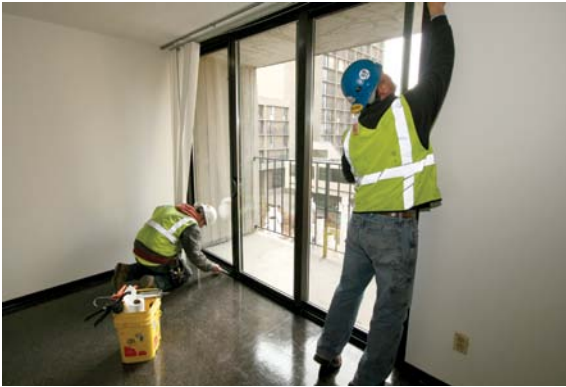
Skilled laborers replaced 2,300 windows and 1,006 patio doors at Riverside Plaza, Minneapolis (right), where exorbitant utility bills, caused in part by 40 years' worth of air and moisture leaks, have been reduced significantly.
